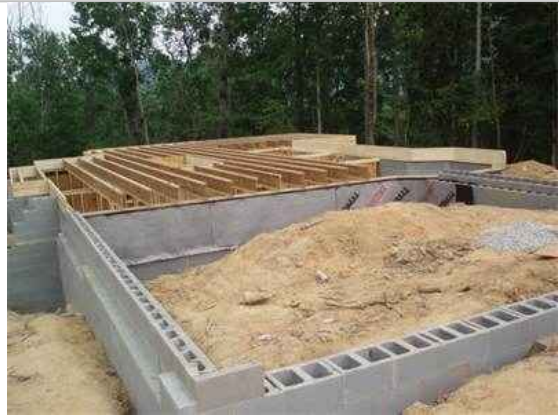
Foundations Rough Carpentry (Labor)
