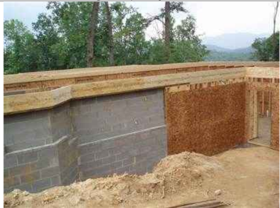
Grading / Backfill Left View
