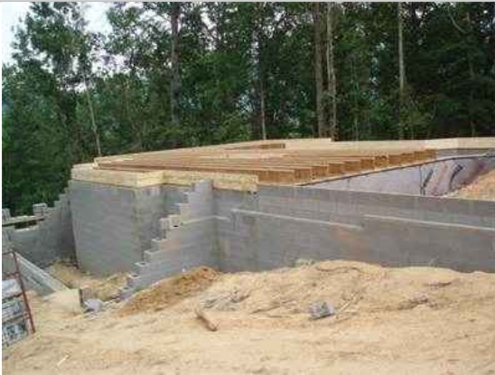
Foundations Block/Retaining Walls
