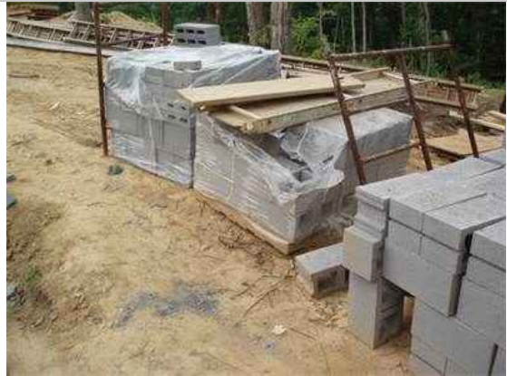
Foundations Block/Retaining Walls
